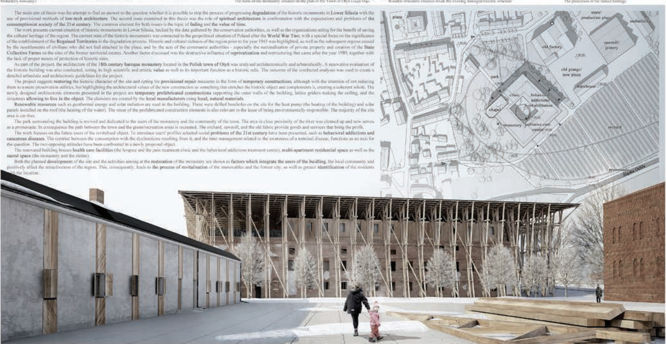
Old garage and main elevation of the main building. Low-tech views of the 18th century baroque monastery. The newly designed architectural elements are temporary prefabricated constructions supporting the entire walls of the building, later grates making the roof and the structure allowing to live in the object. The elements are created by the local manufacturers using local, natural materials.
