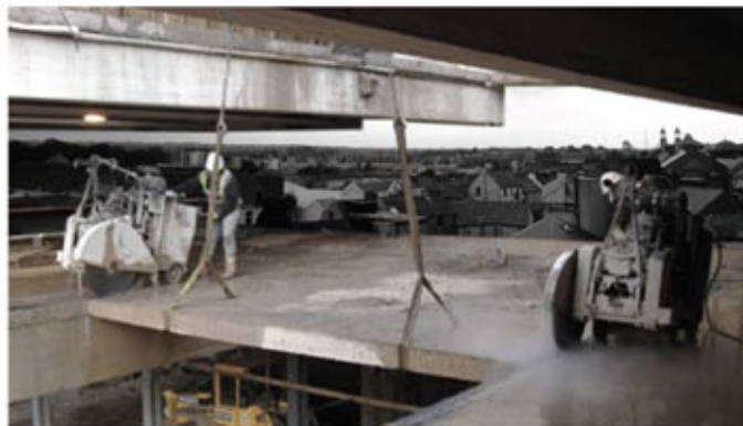
Image portraying the cutting process of concrete which is proposed for the existing car park.
